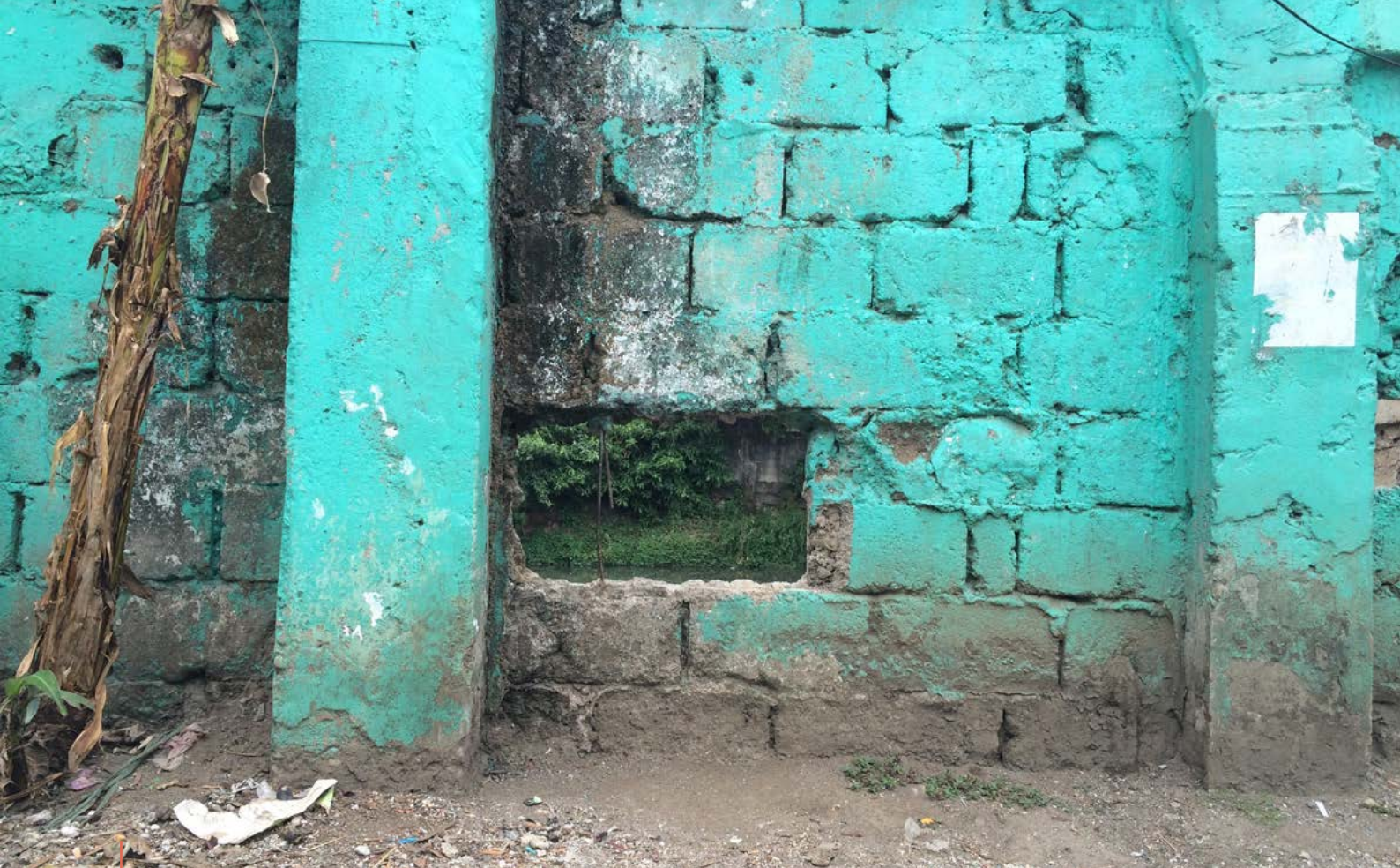
DRR: In order to be able to escape in case of floods, shanty residents knocked holes through floodwalls that separated their homes from the neighbourhood. Photo © Jeremy Harkey
