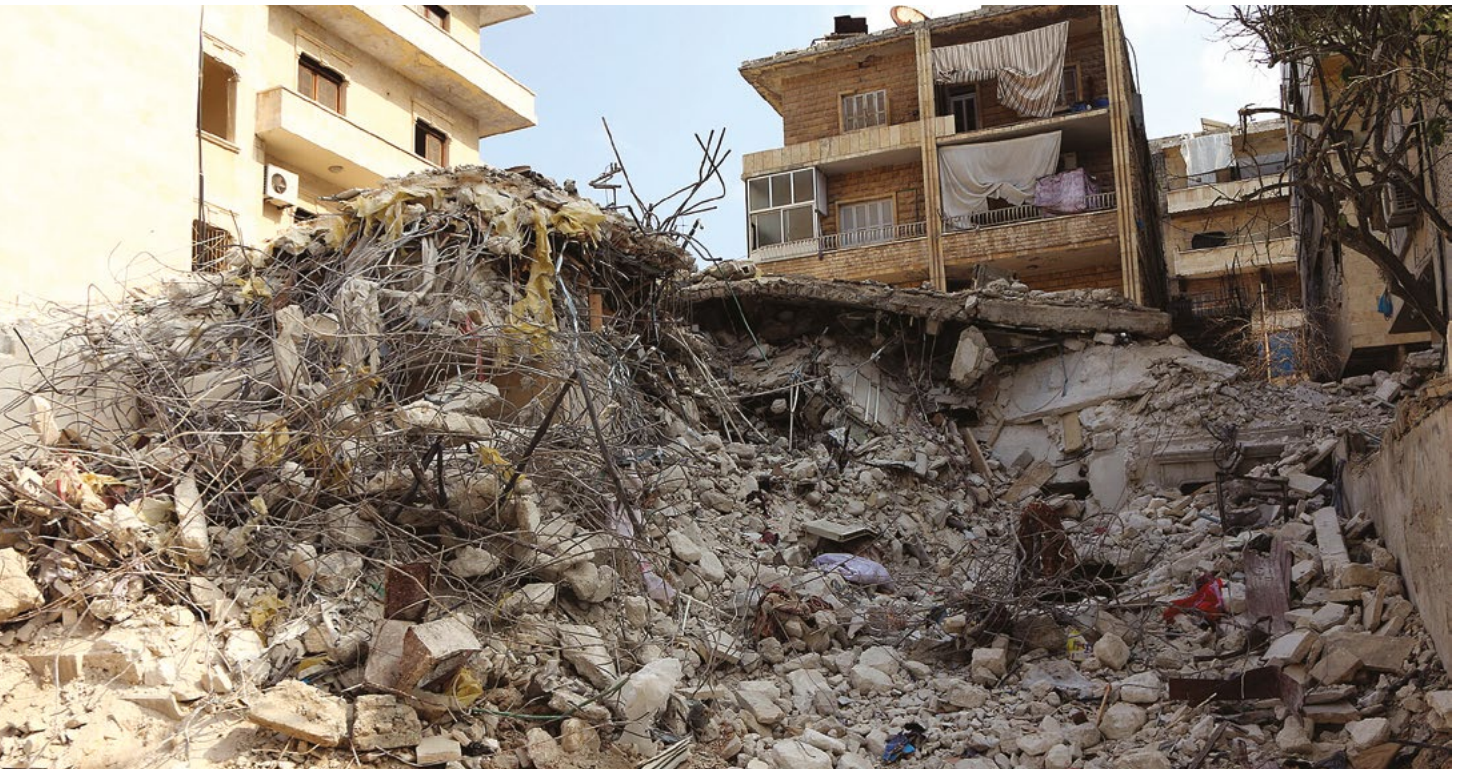
📷 The ruins of a collapsed house in Northwest Syria
