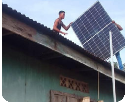
Rooftop solar panels being installed
