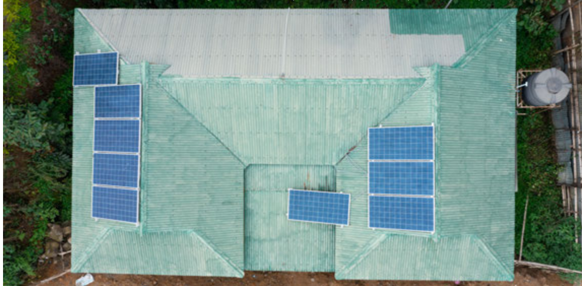
Even in facilities connected to the grid, unreliable power supply can impact service provision
