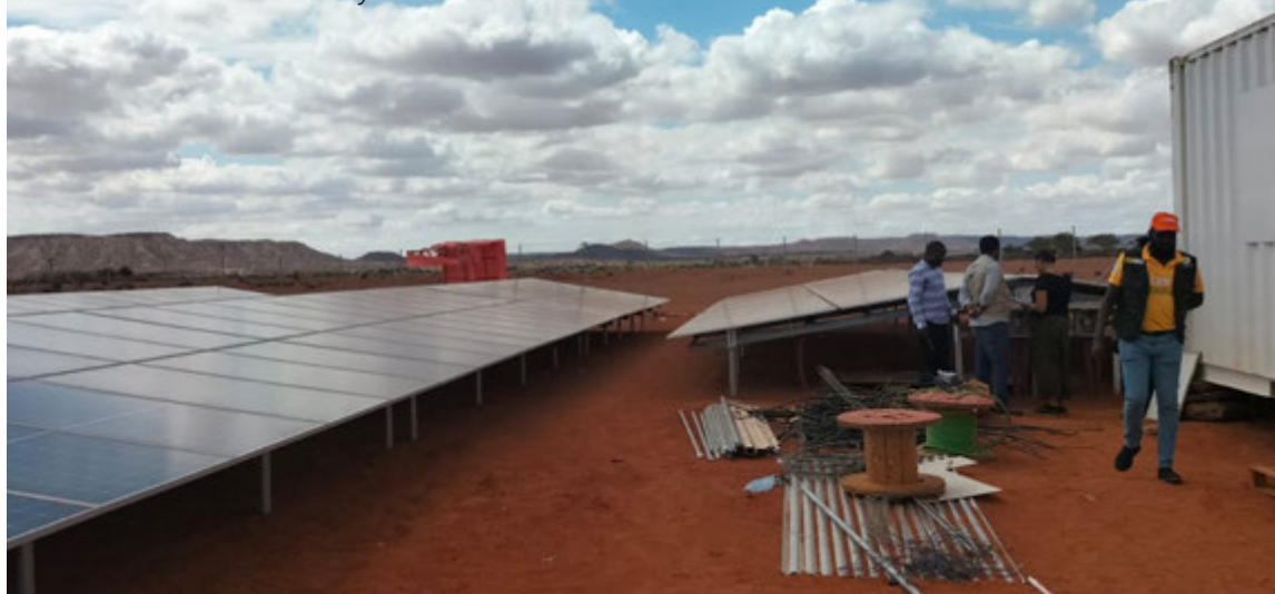
Installation works underway
