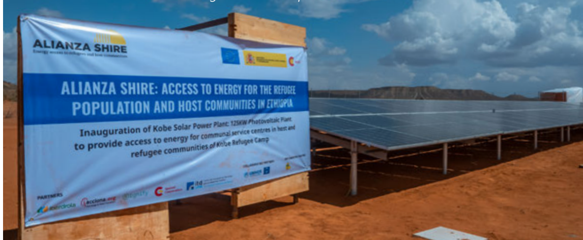
The Kobe Solar Power Plant is inaugurated in Ethiopia
