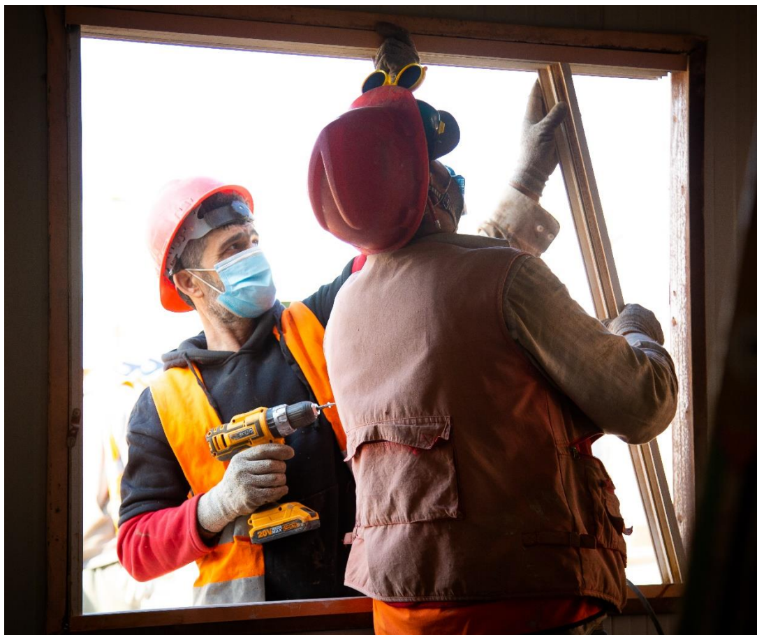
Incentive-based volunteers installing a window as part of NRC's caravan repairs in Zaatari camp, Jordan. Photo: Tina Abu Hanna/NRC
