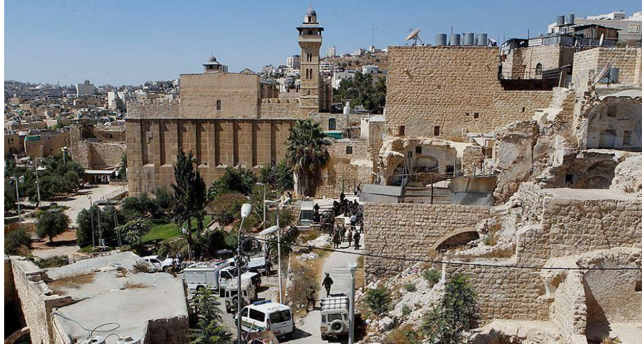
Figure 12: Stopping HRC team during restoration works
