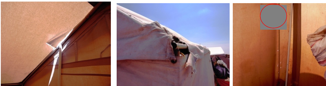
Pictures of tents: damage and tears in canvas (in Arafat settlement, Galkaiyo)
