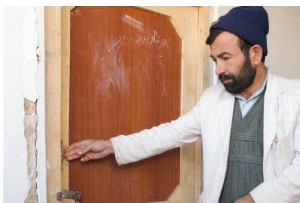
Doors fitted in NCR shelter
