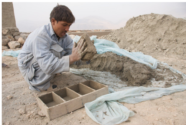
A beneficiary builds mud bricks for his house in Chamtala LAS
