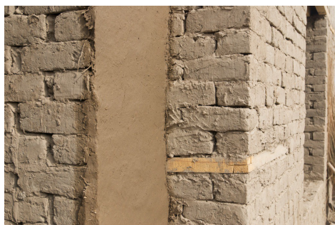
Timber triangles inserted in the wall of a house
