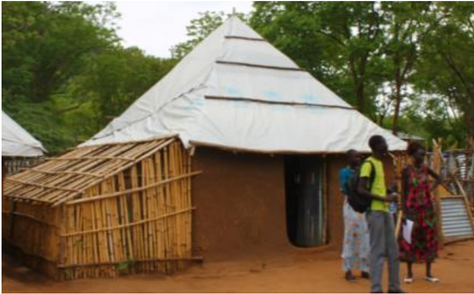
Picture 1 - Sample shelter constructed in Kule camp, Gambella. See added 'extension'
