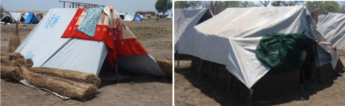
Picture 4: A simple, ‘A’ frame emergency shelter in Leit-chuor & Tierkidi camps, Gambella
