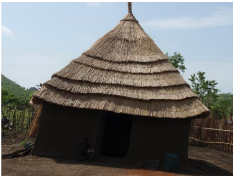
Picture 2 - A tilting Tukul Shelter in Zone D, Tierkidi Camp, Gambella.
