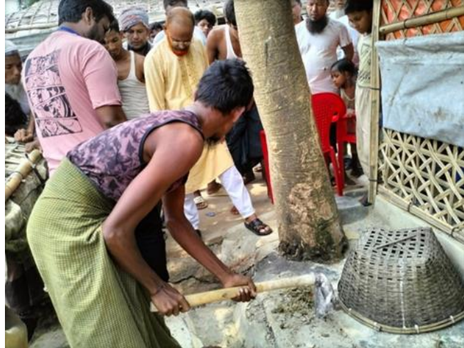
Access points being restored. ©NRC
