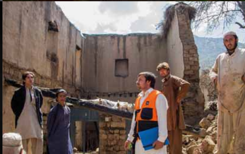
NRC's field engineer is monitoring the community based shelter construction of a damaged house in Kurram Agency, Pakistan. Photo: NRC Pakistan/Shahzad Ahmad
