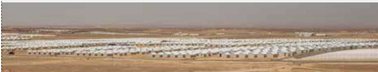
HARSH CLIMATE. NRC has developed a new type of shelter suited for the extreme conditions of the Jordanian desert, where the Azraq refugee camp is located. Photo: NRC/Shahzad Ahmad
