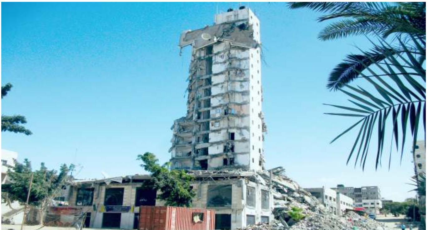
The Italian compound in Gaza City was destroyed in the final days of the most recent military escalation. Residents have been forced to seek alternative accommodation, many resorting to temporary rental arrangements, 2014. Photo: NRC.
