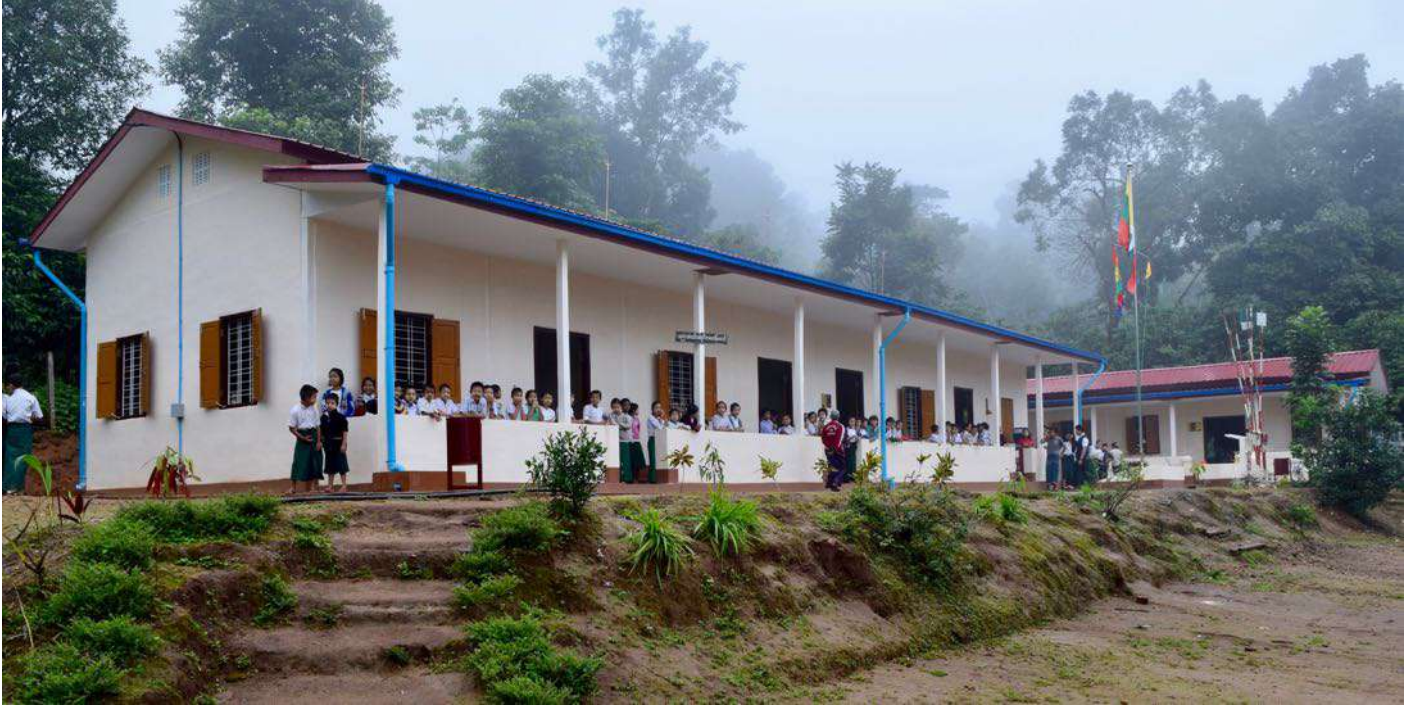
Newly renovated and constructed school in Za Le village, Kayin.
